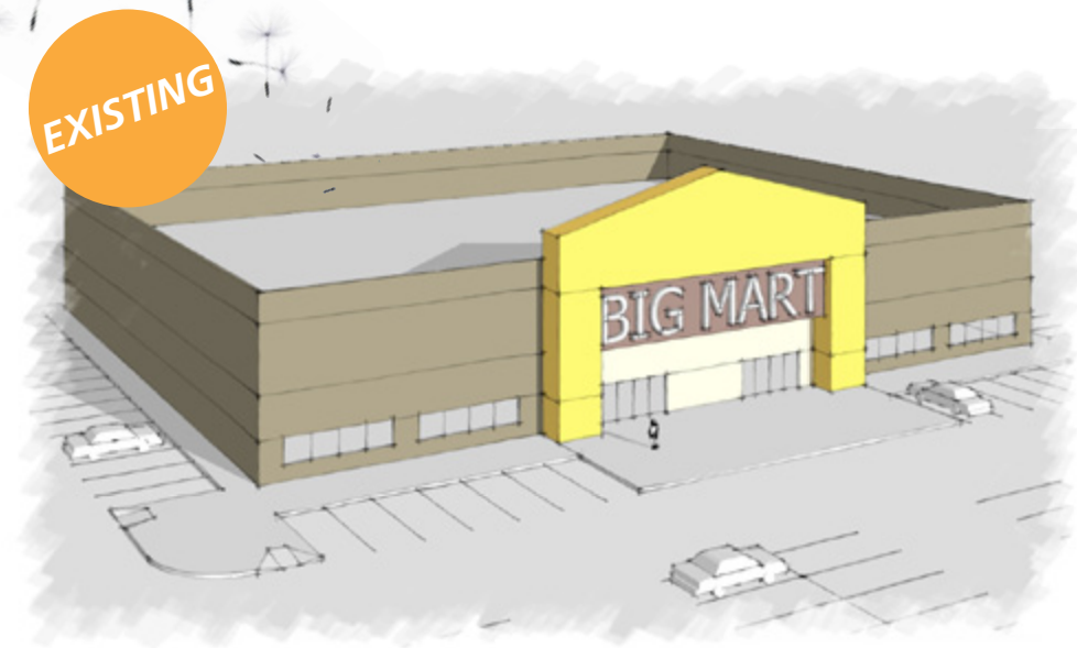
The classic big box retail sits vacant awaiting vandalism, deterioration, and eventual destruction. This is the story for many big box retailers around the country.
